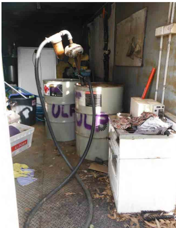
Photo 13 - 44 Gallon Drums of Unleaded Petrol with storage container adjacent to Jet Fuel Tank.
