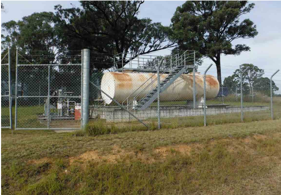
Photo 11 - 30000 L Jet Fuel AST (Within AEC38)
